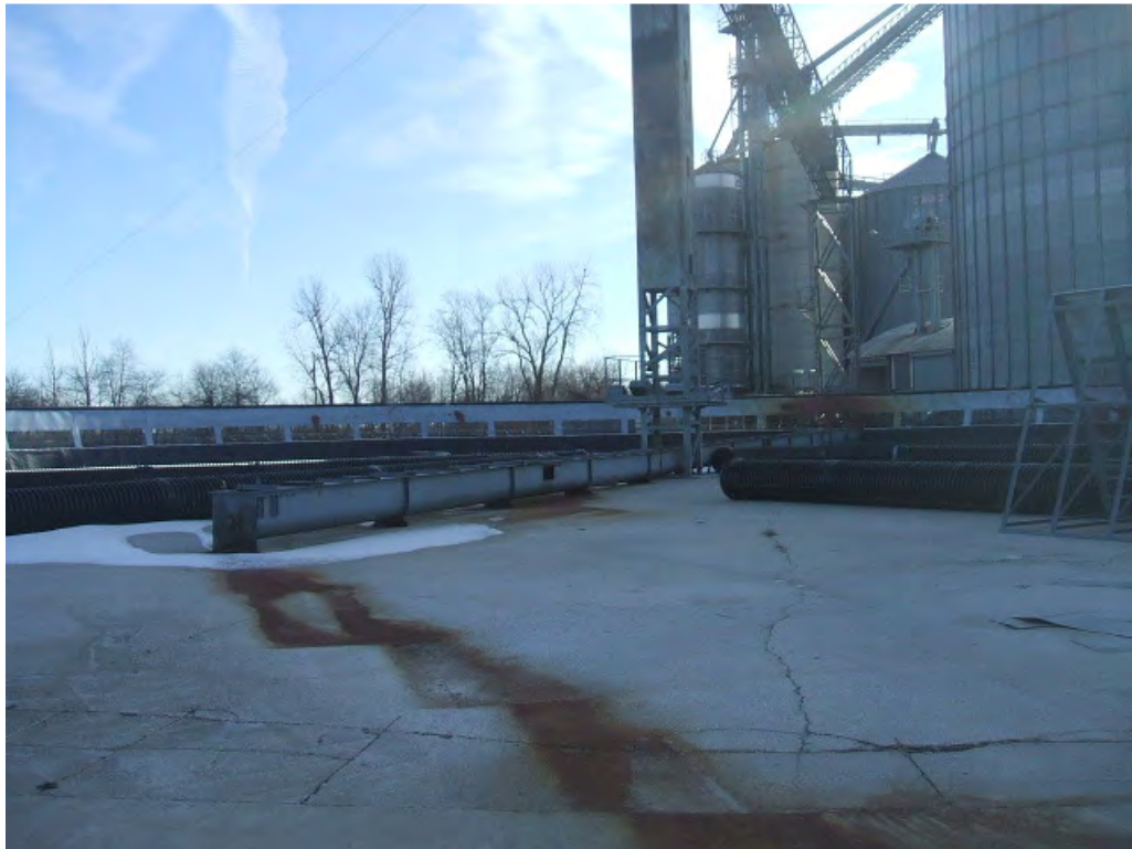
Photo #20: View of the circular grain storage area.
