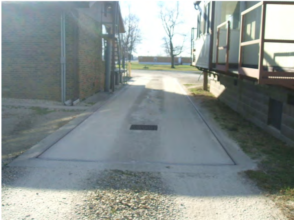
Photo #10: View of one of the weigh scales with three floor drains.
