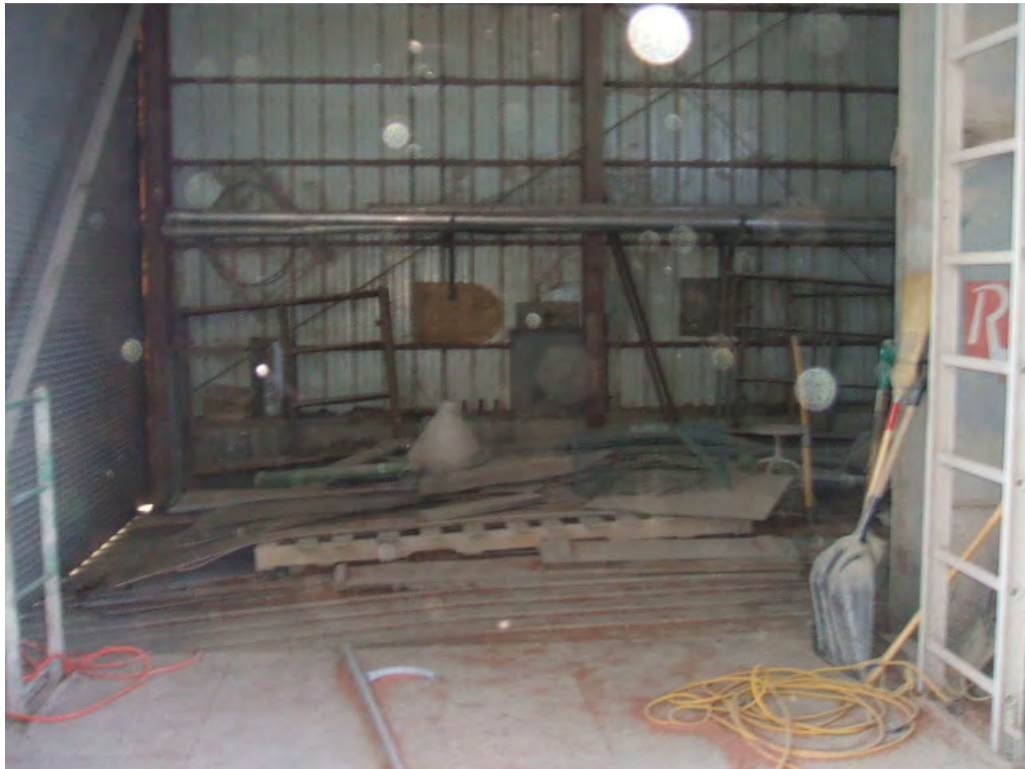
Photo #16: View of storage area in the steel framed building.
