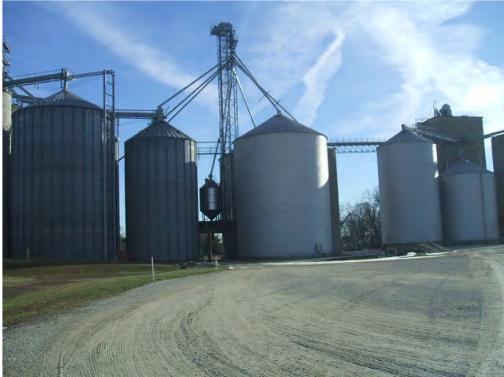
Photo #5: View of the silos facing east.
