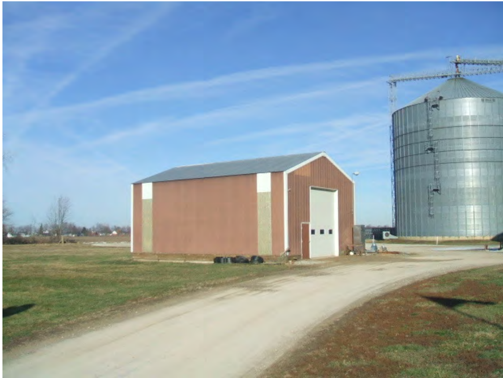
Photo #13: View of the pole barn facing northwest.
