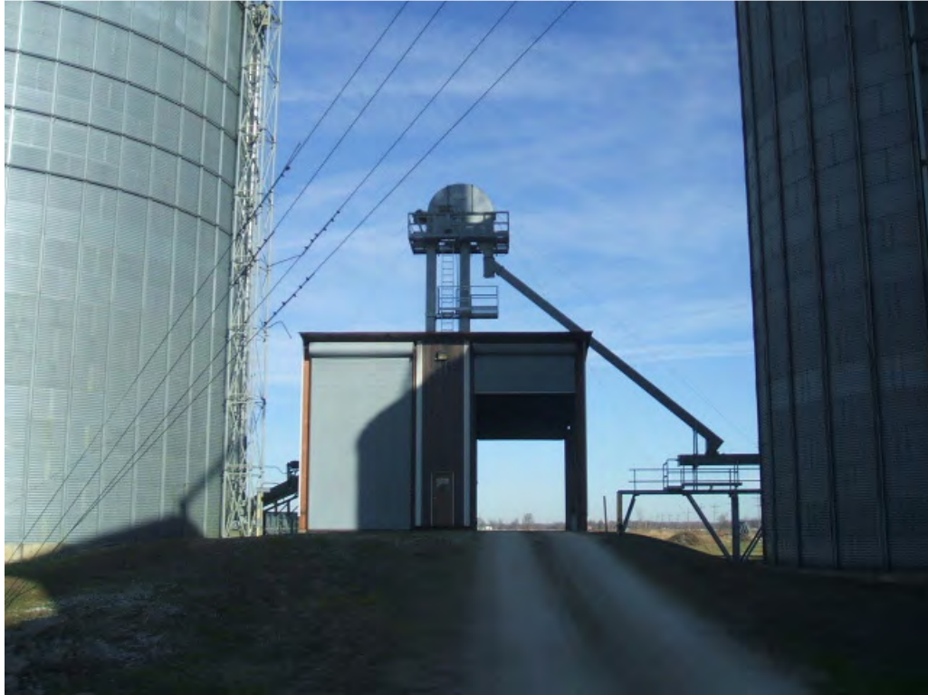
Photo #15: View of the steel framed building.
