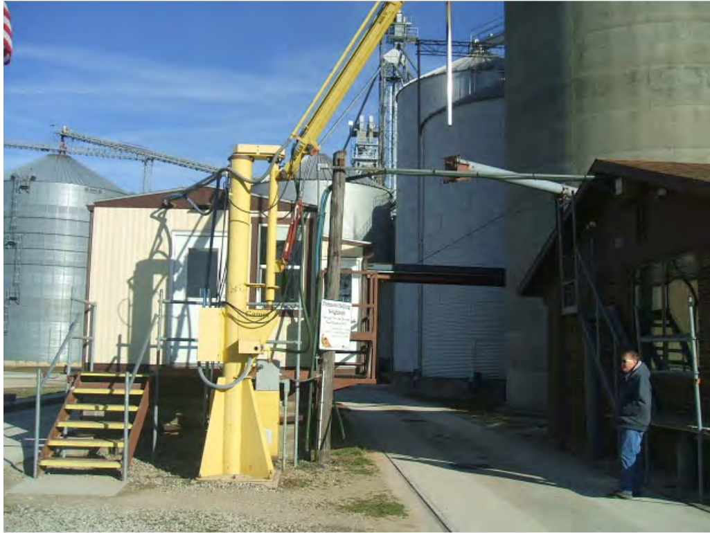
Photo #9: View of the hydraulic truck probe.
