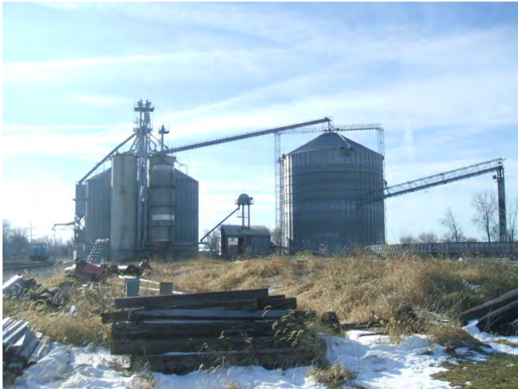
Photo #4: View from the northern gravel road facing south towards the silos.
