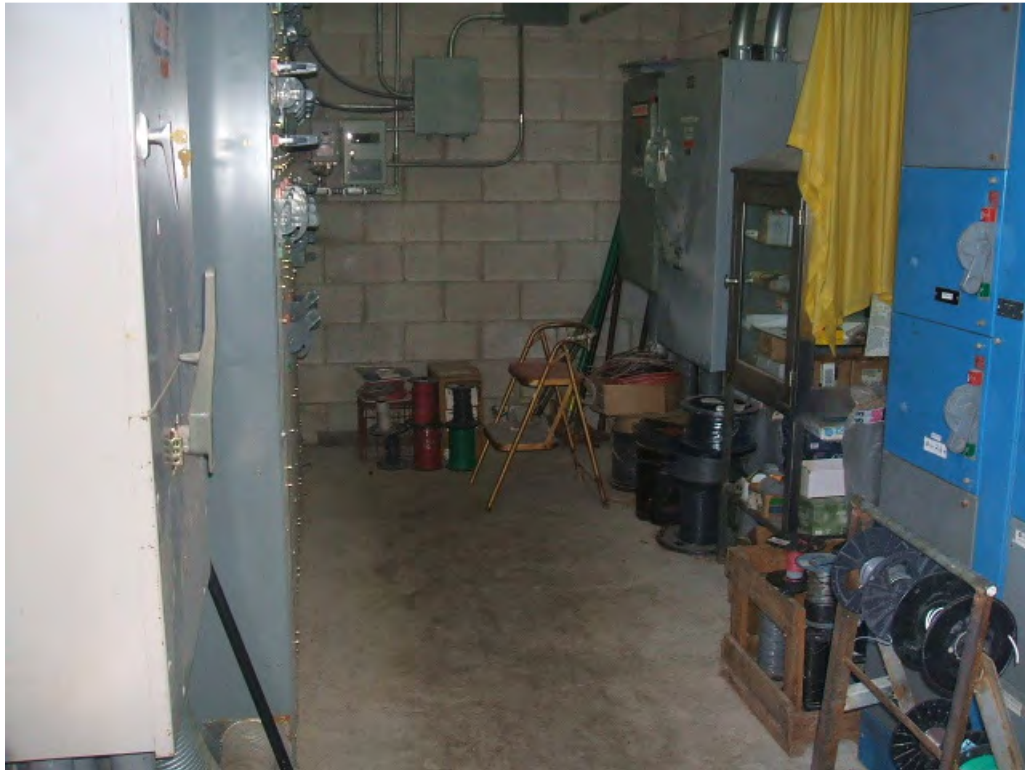
Photo #17: Interior view of the utility/storage building.
