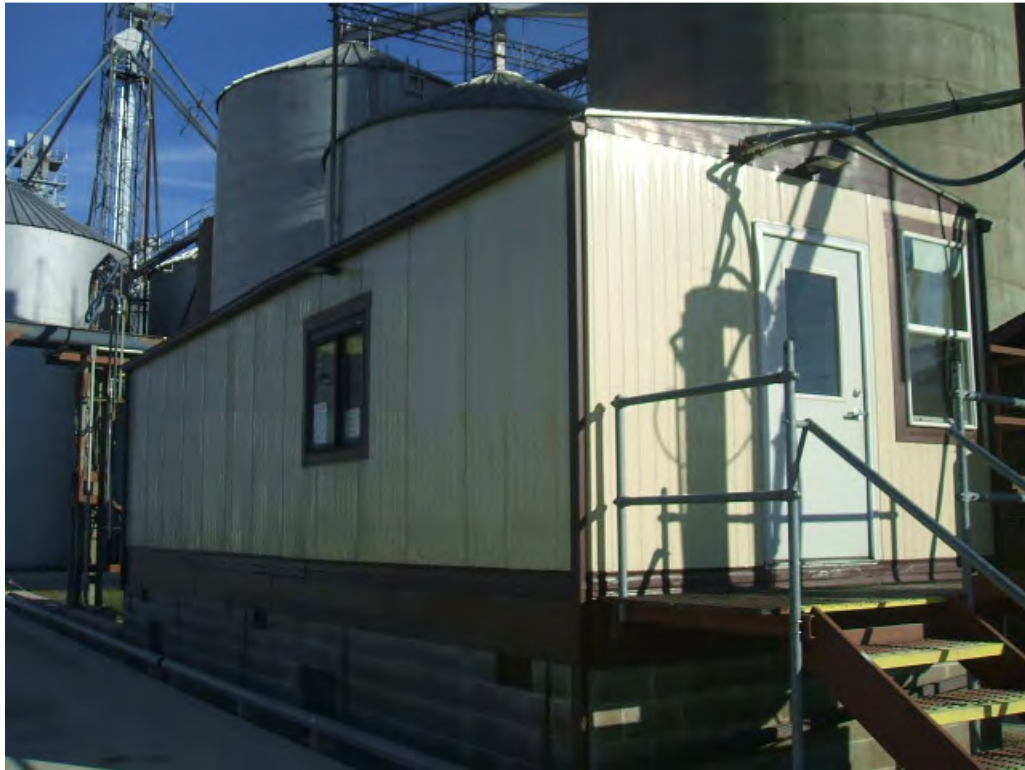
Photo #7: View of the weigh-in trailer.
